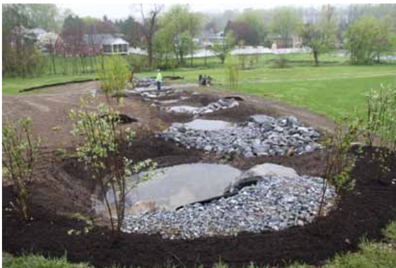
The completed RSC project
