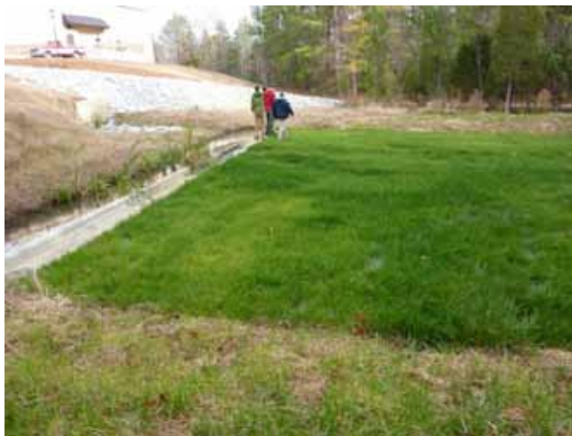
Figure 1. Example urban filter strip (Photo courtesy of Ryan Winston, North Carolina State University).
