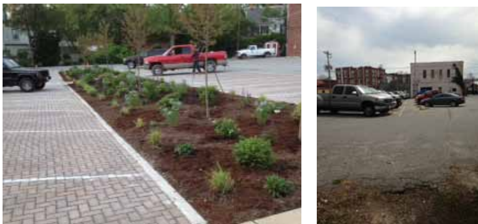
Figure 1. Town of Onancock permeable parking lot site before (left) and after (right) installation
