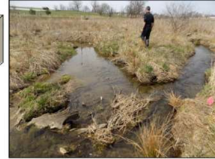
Legacy sediment removal Big Spring Run, Pennsylvania, USA
