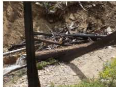
Unanchored introduced logjam Black Hollow, Colorado, USA
