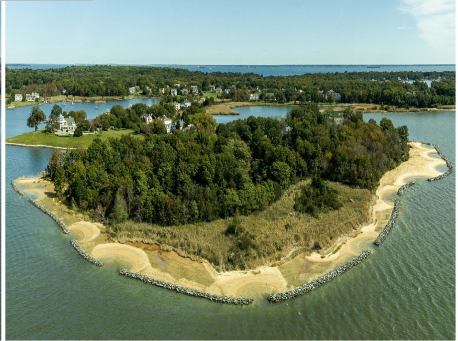
Immediately After Construction – October 2020
