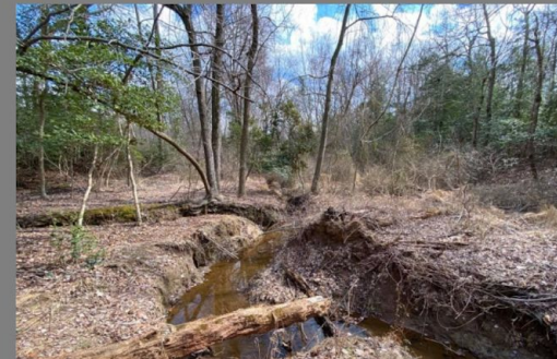
Beards Creek/Annapolis Landing Stream Restoration Awardee: Arundel Rivers Federation
